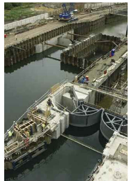
Work in progress in the Prescott Channel
